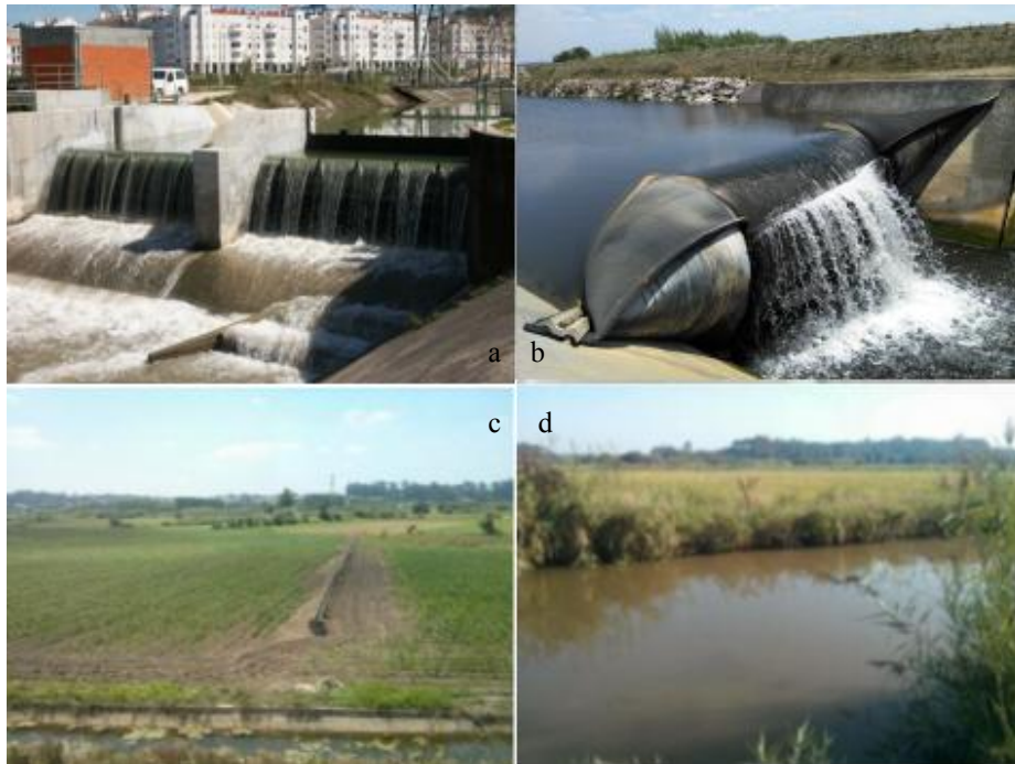
Fig. 3. View of the irrigation district: a) Arrabalde weir (to supply sectors C1 and C2); b) inflatable weir (to supply sector C7); c) secondary canal and surface irrigated field (sector C7); d) main drain ditch (sectors C4 and C5).
